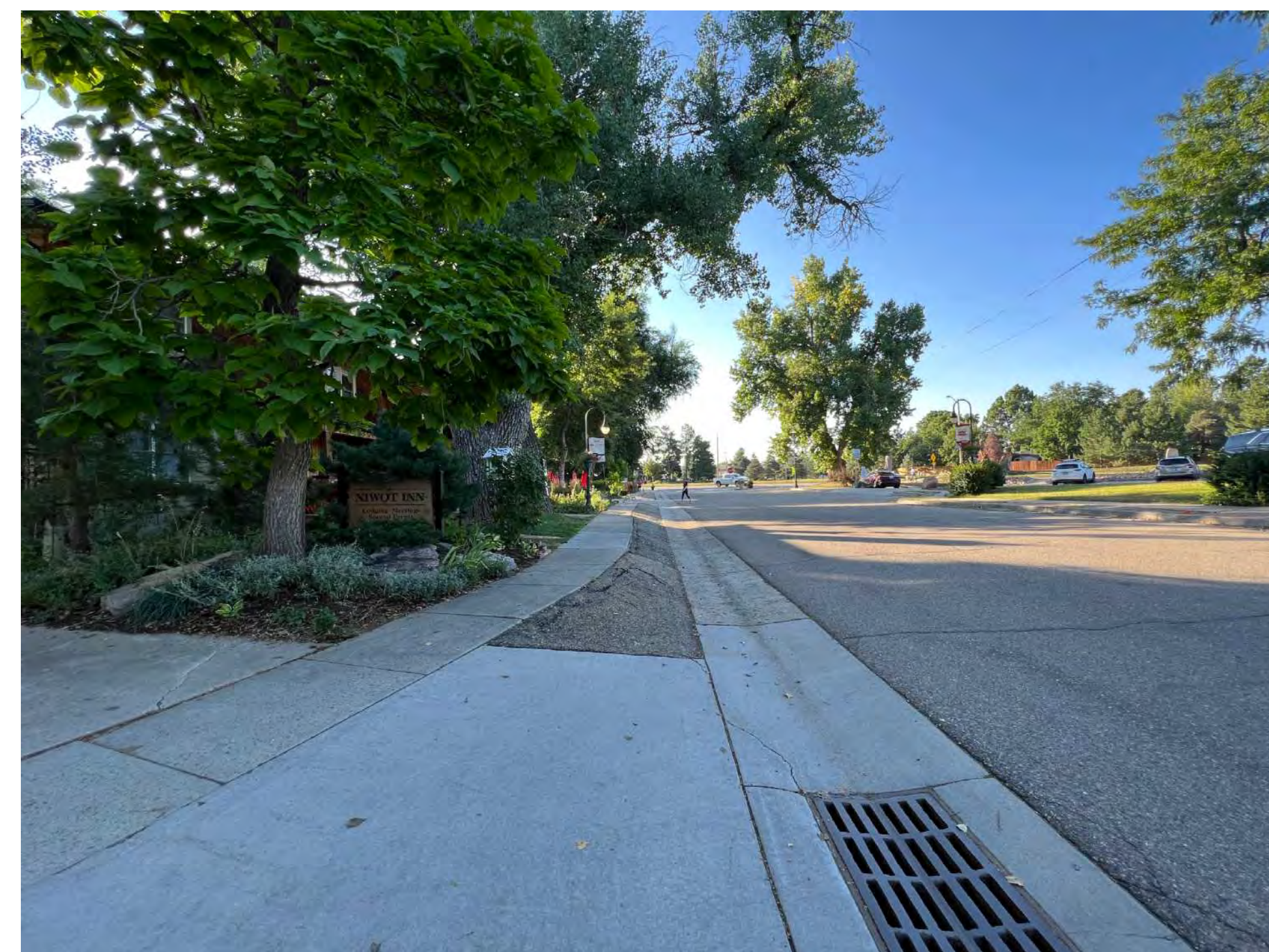
In some sections the sidewalk narrows and there is a steep transition down to the street elevation creating a dangerous condition for pedestrians.
