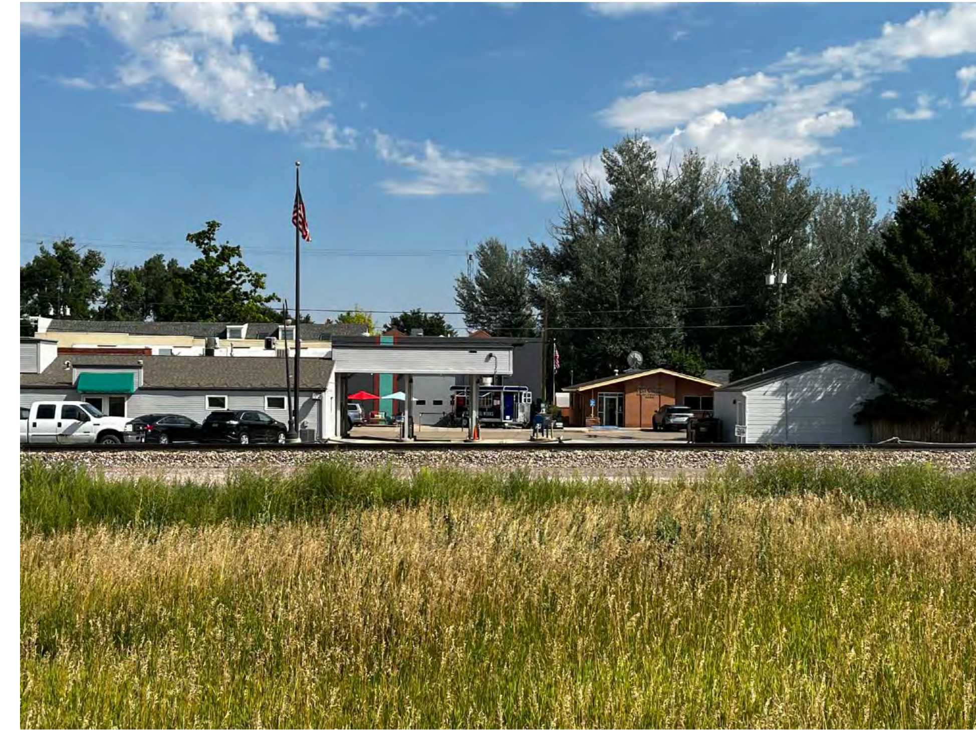
The western facade of the bank, its parking lot and drive-up from Diagonal Highway is an important opportunity to enhance and improve the first impression of Niwot.
