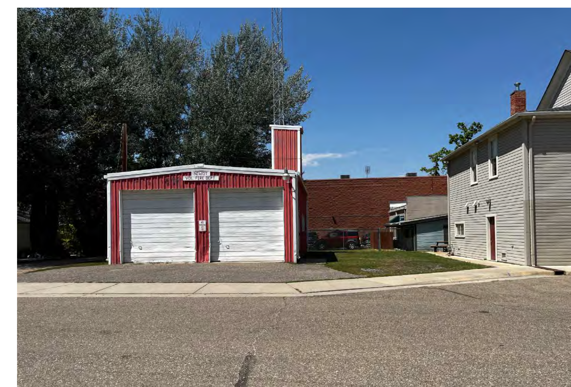
The metal building located at the back of the Hall occupies precious space that could potentially function as an outdoor area for the Hall events expanding its capacity and value.
